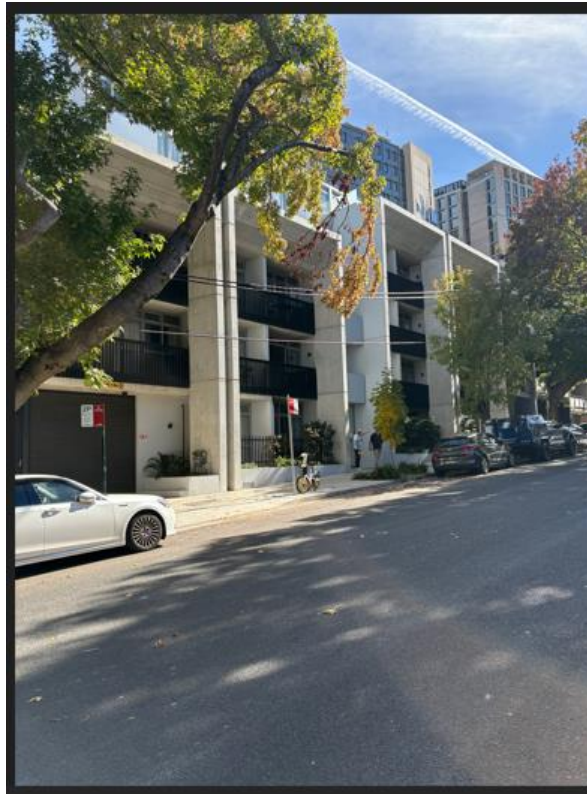
Figure 1: 16 Cope Street, Redfern, viewed from the south-east
